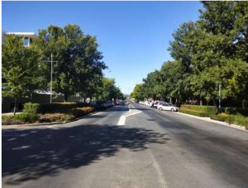
Figure 2-6: Looking south along Wodonga Place towards Smollett Street
